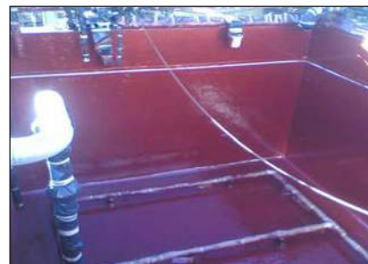
ARC CS4 final application
