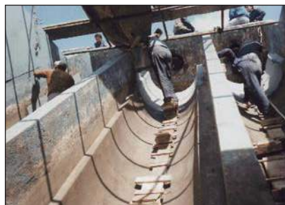
ARC 791 applied to properly prepared surfaces
