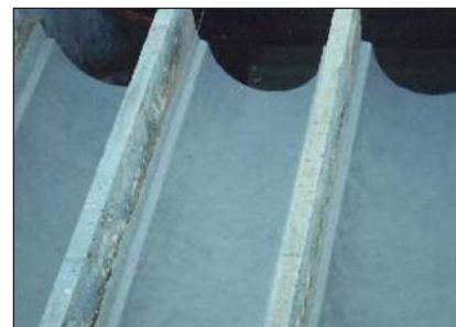
All three pump troughs coated with ARC 791
